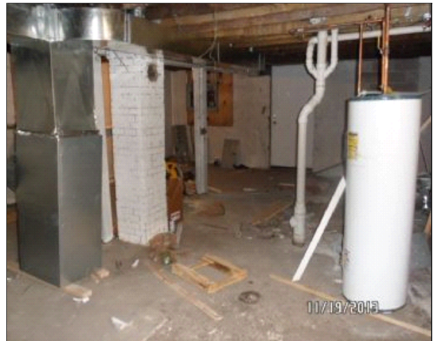
Furnace and Hot Water Heater for unit 1
